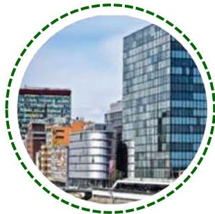
Building Utility & Cooling
